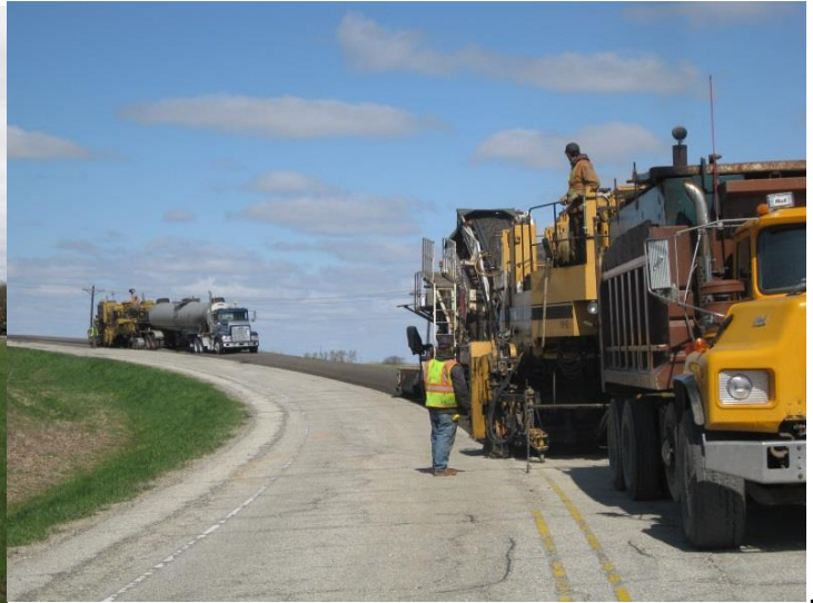
Adding Binder, Placing, and Compacting
