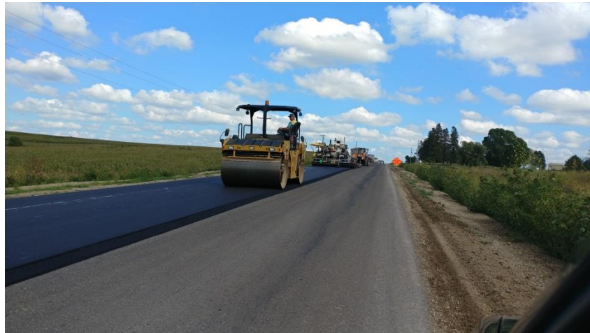
Additional Hot Mix Asphalt (HMA) lifts over the CIP (Golden Road 2017)
