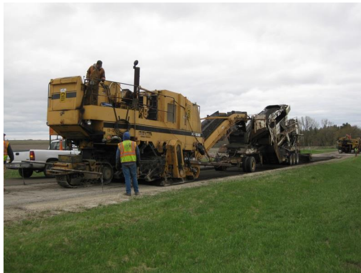
Additional Hot Mix Asphalt (HMA) lifts over the CIP (Golden Road 2017)
