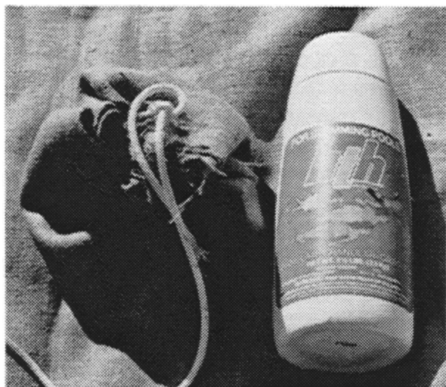
Fig. 1. Cloth sack filled with powdered chlorine is ready to be lowered into the well.
