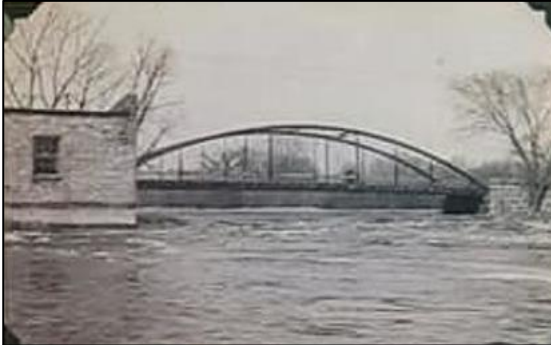
This 1936 iron bridge stood until 2003 at which time a new concrete bridge was constructed.
